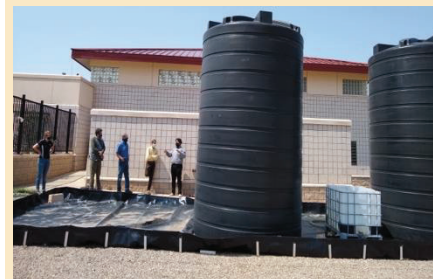
Fig. 2. Produced water storage tanks in BGNDRF for pilot projects
